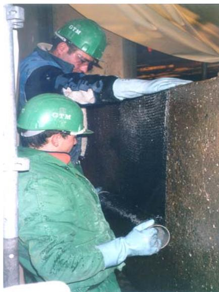
**Figure 3** Carbon-fibre sheet material and its installation
